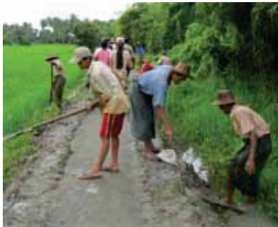
Cash-for-Work programs include footpath construction.
