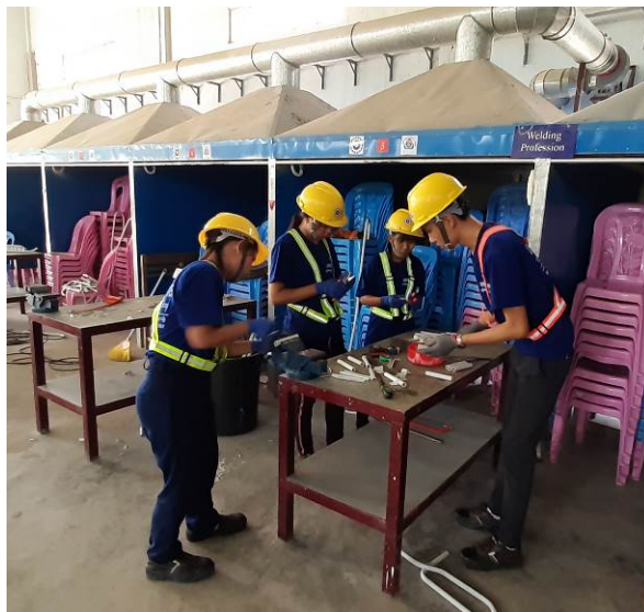
Male & female students - learning pipe installation and trucking in the Electrical Wiring Course
