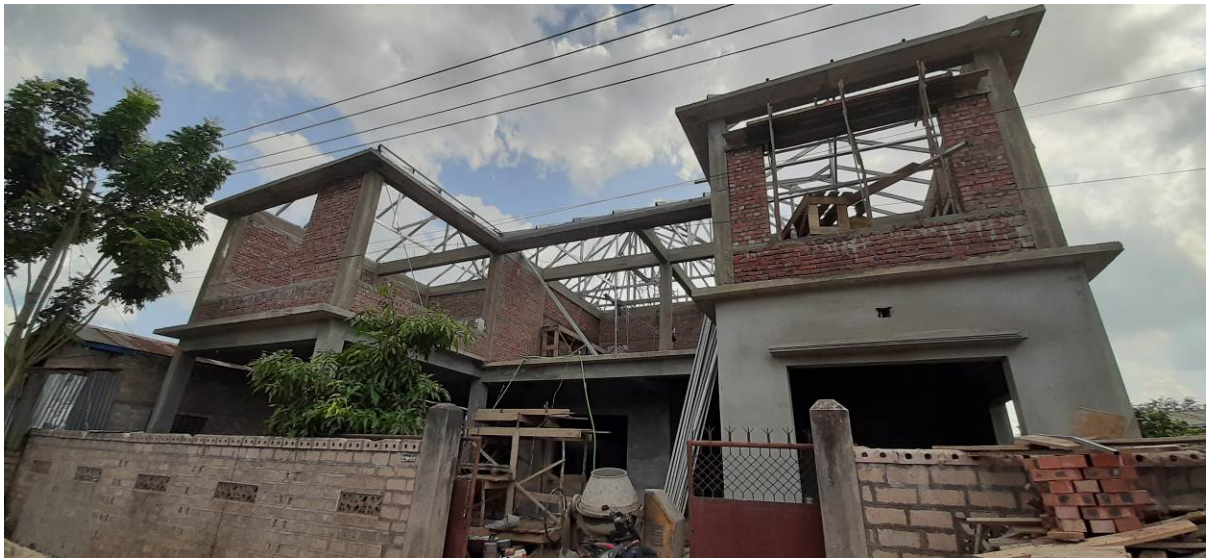
Un-finished construction site in Lashio
