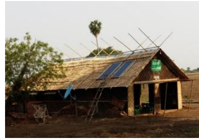
House in rural Myanmar equipped with solar panels
