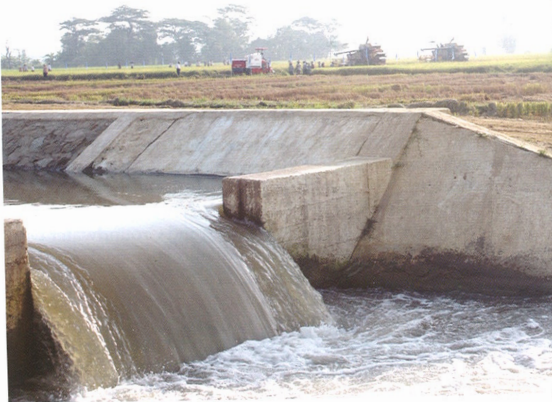
Constructed River Water Pumping Projects
