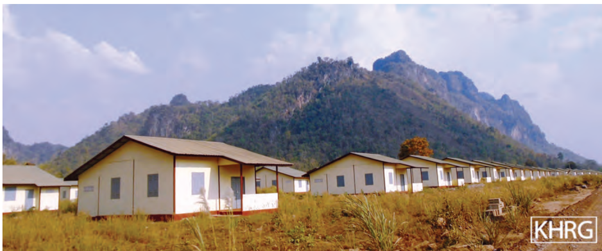
This photo was taken on February 26 th 2017 in the Lay Hpa Htaw repatriation site, Noh T’Kaw (Kyainseikgyi) Township, Dooplaya District. They show the houses that were built for the repatriated refugees right after their construction. Even at that time, an interviewee from nearby Deh Ther Pler pointed out that the lack of farmland around the site will create problems for future returnees: “There is [we will get] only one house without land to farm for our livelihood. Therefore, where will we get food if we return to that area?” [Photo: KHRG]
